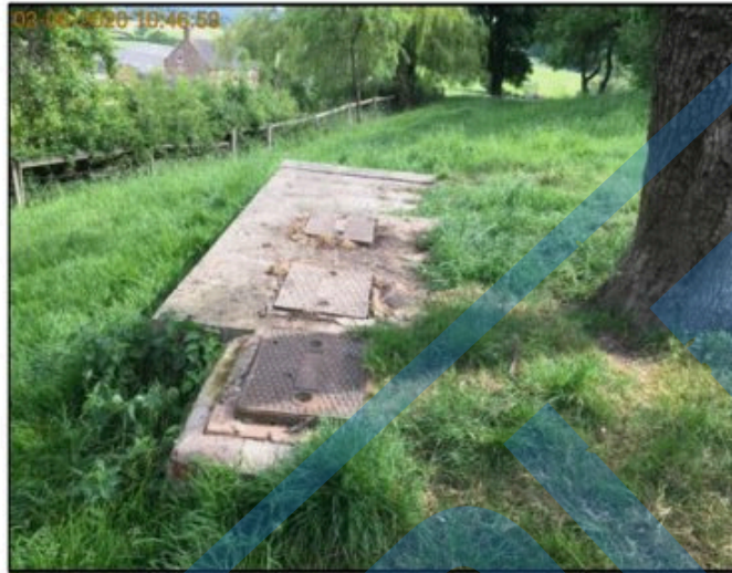
Photograph of the general area of the tank:
